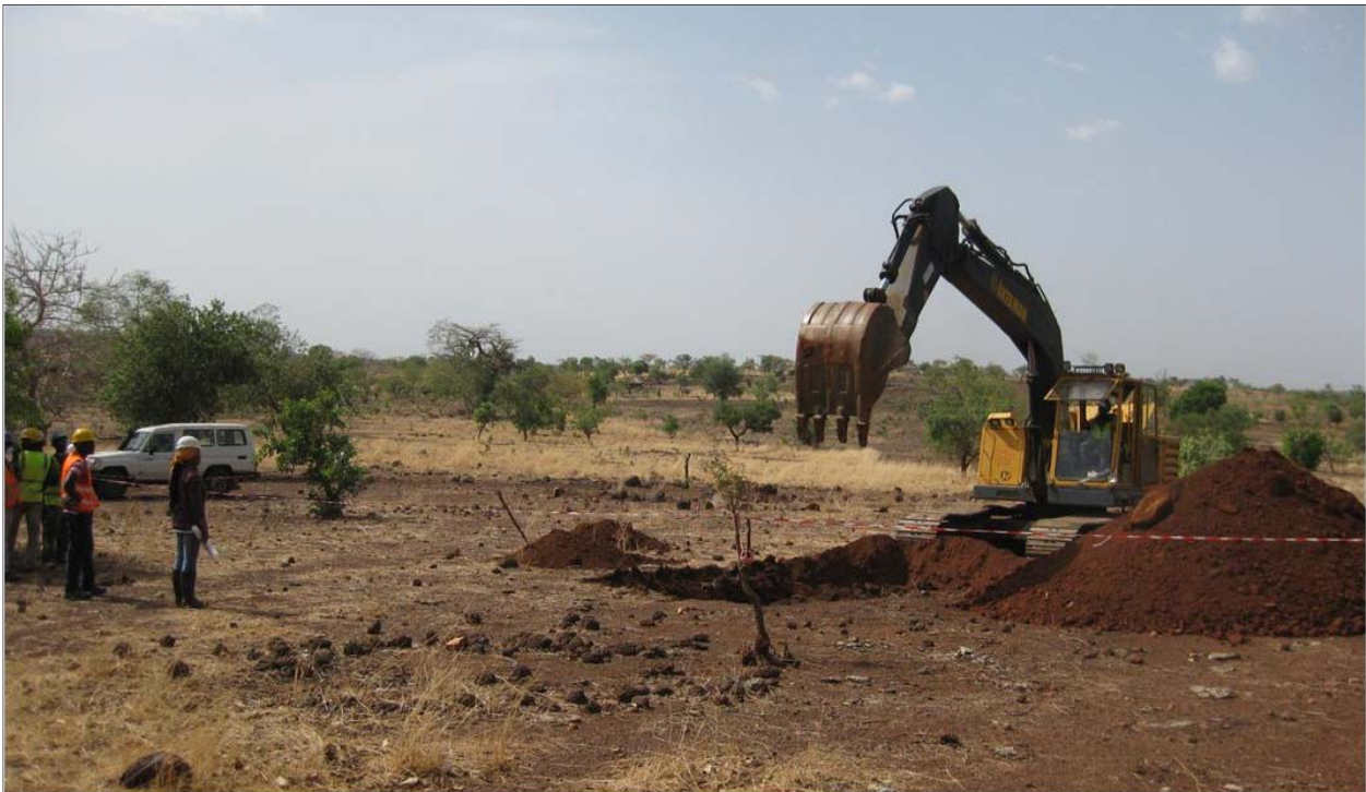
Natougou Project - Excavating test pits for geotechnical assessment of process plant site.
