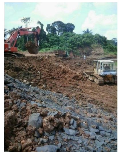
Figure 3 – Removing further Overburden
