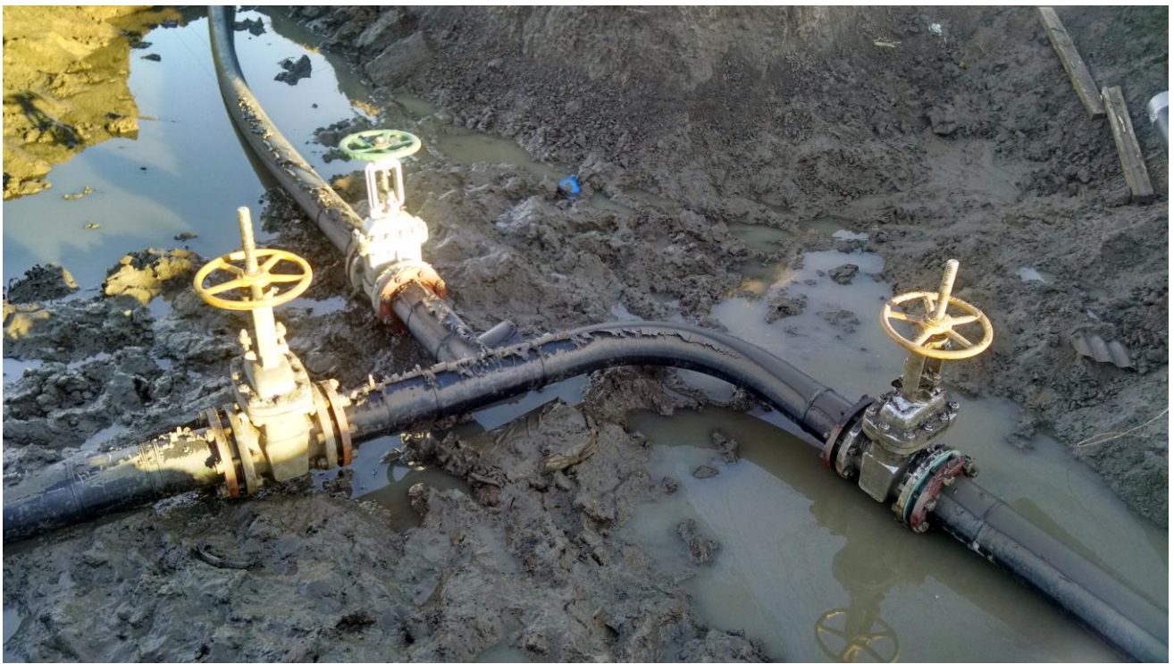
Figure 5: Infrastructure plumbed to manage flow bi-directionally, ultimately enabling gas delivery to either sales point
