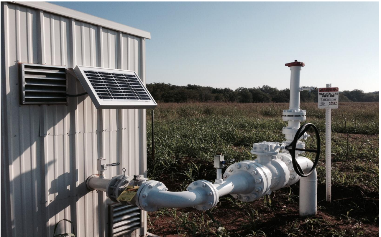
Figure 3: Gatherer's gas line immediately behind AusTex's check meter.
