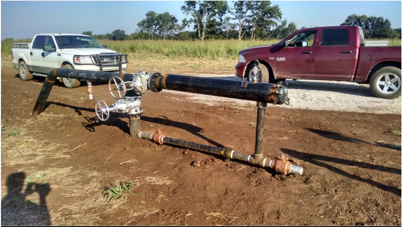
Figure 4: Pig receiver – these are arrayed across our lines to ensure they remain clear and available.
