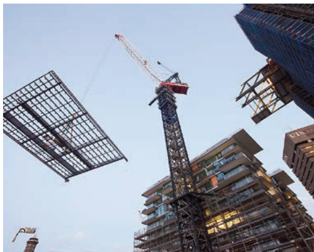
Lifting the heliostat into place during construction of One Central Park in Sydney
