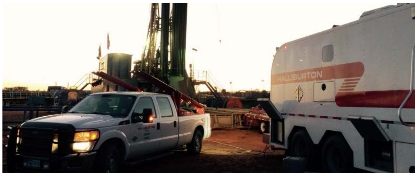
Logging of the Hope Boles PU1 well within the Capitola Oil Project
