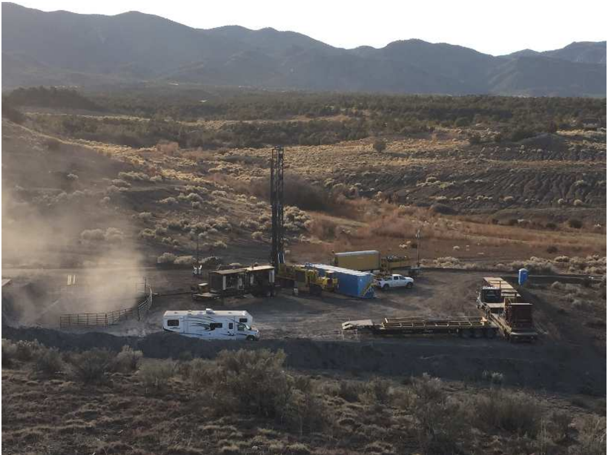
C 18 #3 WELL PATHFINDER PROJECT. FREMONT COUNTY, COLORADO, USA.
