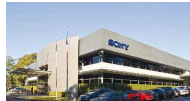
Macquarie Technology Centre
