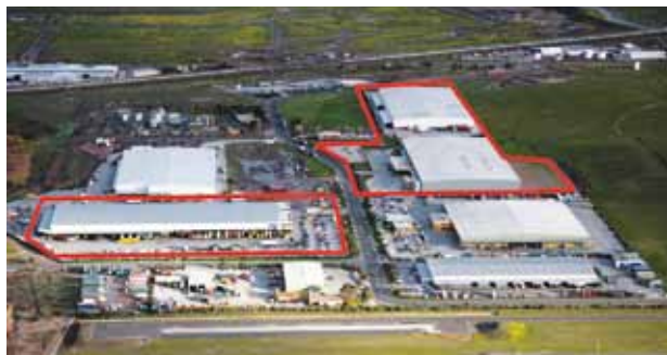
Toll Business Park
