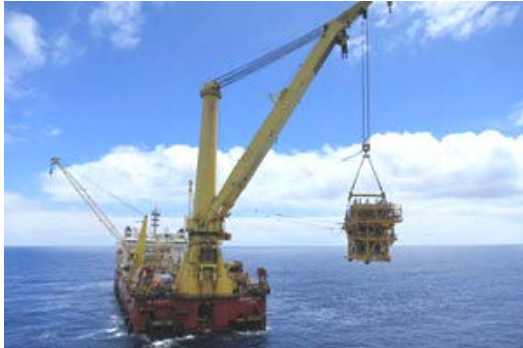
Sapura 3000 heavy lift vessel with Compressor Module suspended
