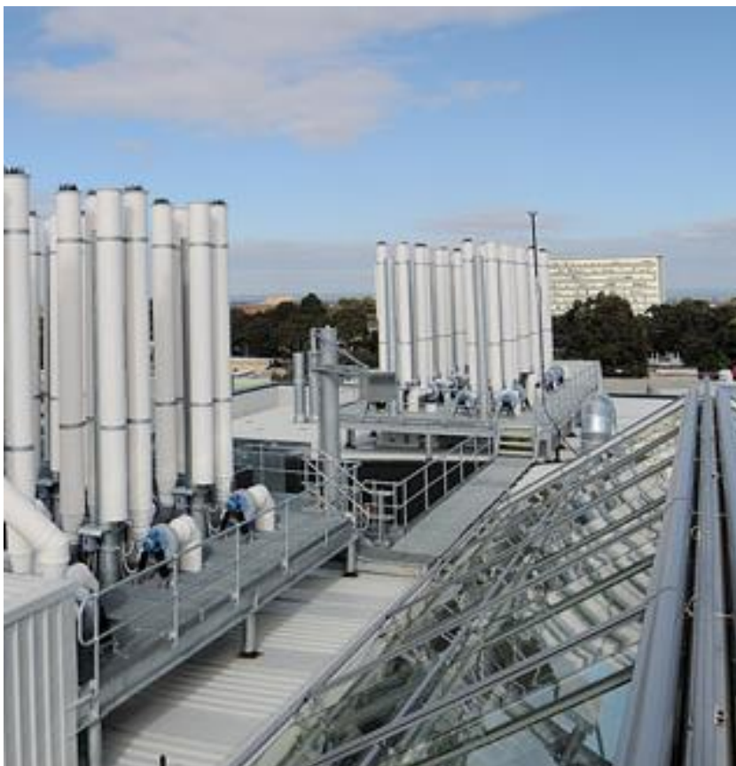
150 exhaust fume stacks were installed on the Monash University, New Horizons Building.
