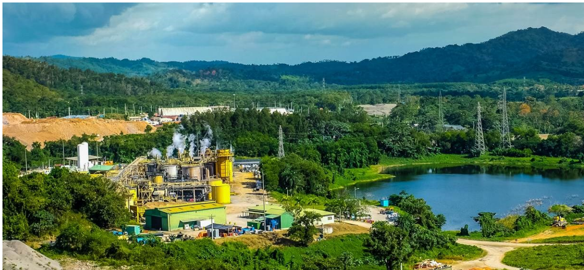
Las Lagunas Albion/CIL Process Plant
