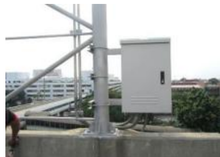
Figure 8: Control Box at each reader site that concentrates the data prior to transmission over GPRS
