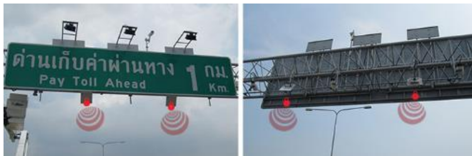
Figure 7: Freeway site in Bangkok showing LPR Camera, CCTV and RFID Reader
