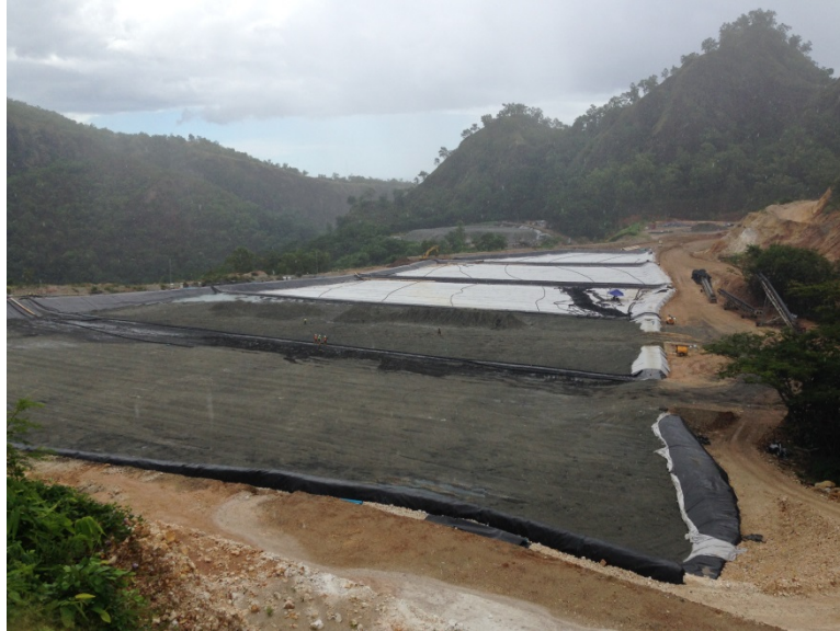
Image 2 – GPLP lined and Cell 1 bedding layer complete
