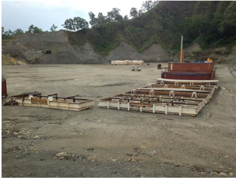
Image 5 – SX-EW plant site with Whim Creek settler tanks in the foreground
