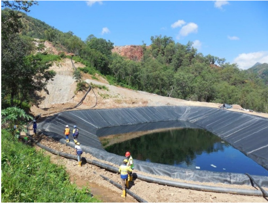
Image 5 : Newly completed Intermediate Leach Solution Pond ready for use
