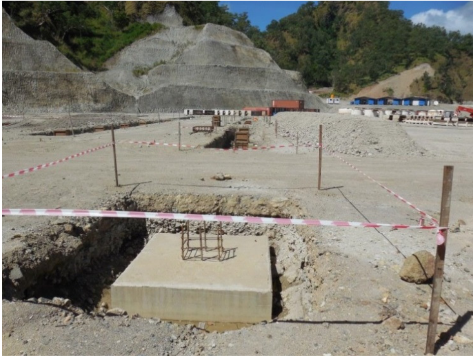
Image 1 : 25,000 tpa copper cathode SX-EW plant concrete footings
