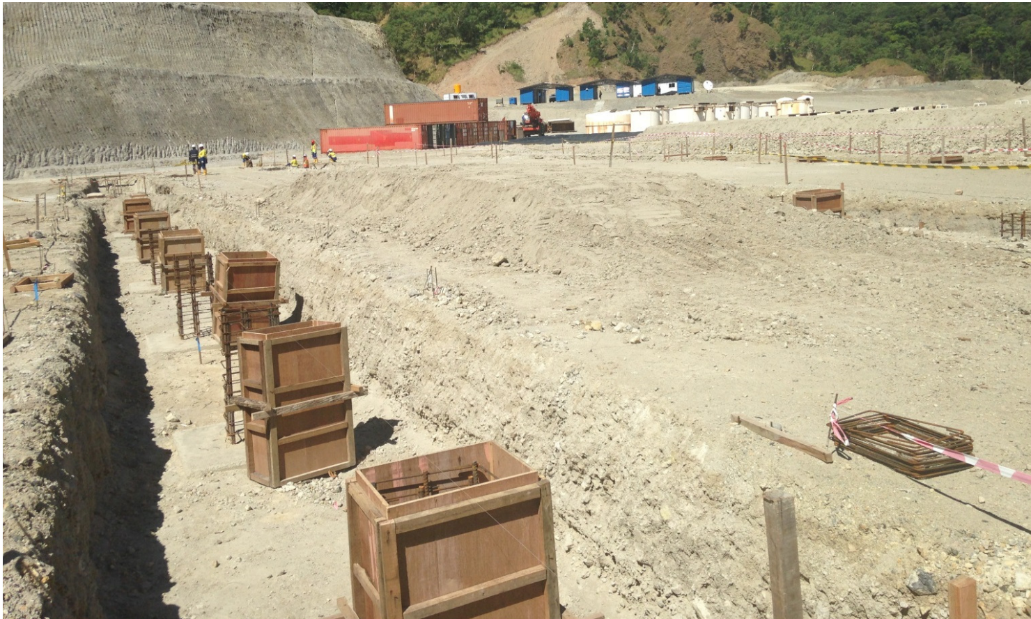
Formwork for footings on the plant site
