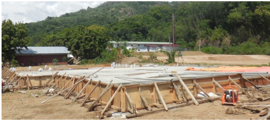
Image 11: New camp mess concrete pad
