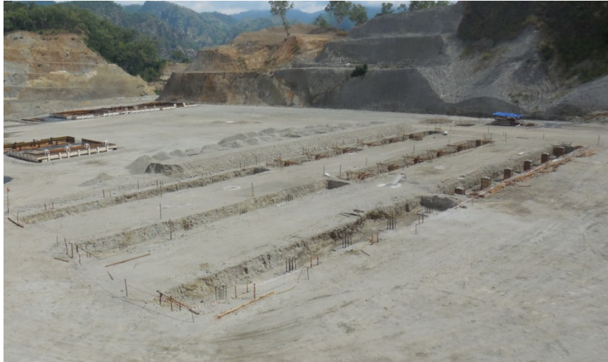
Image 10: View across 25kt Plant concrete footings
