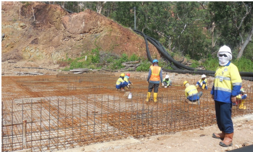
Image 4: Formwork for the concrete pour for the new GPLP Staging Tanks
