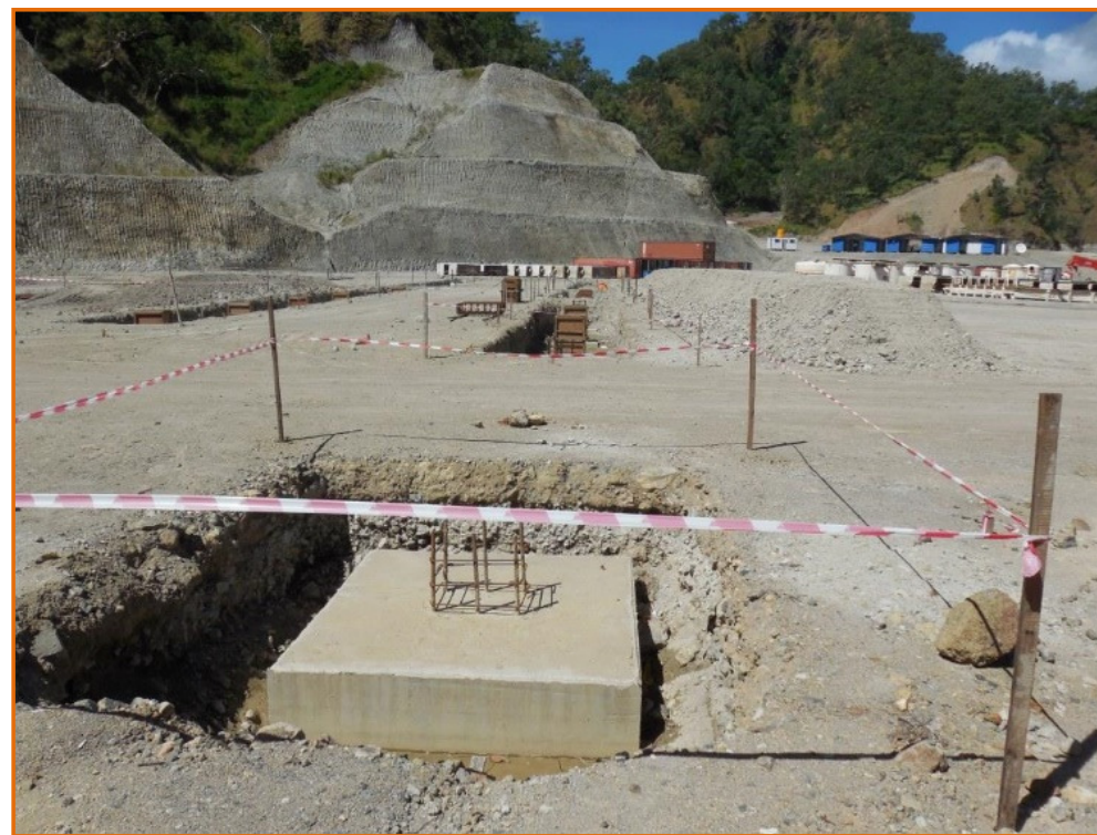
Concrete footings on SX-EW plant site
