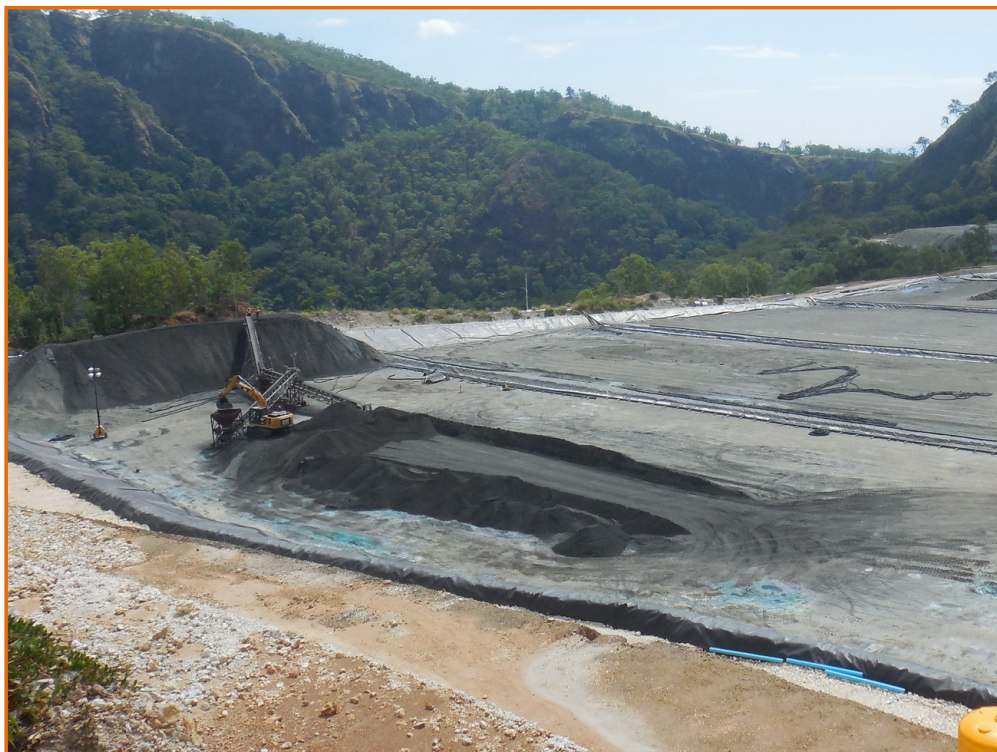
Stacking the Gold Pit Heap Leach Pad
