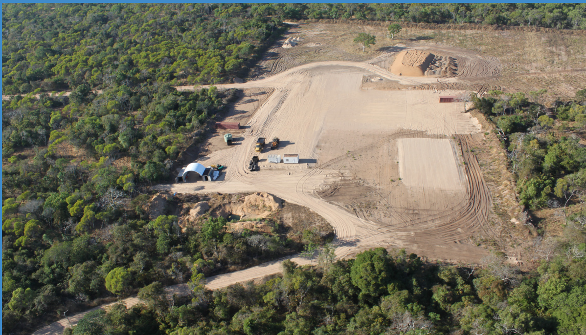
FIGURE 2: Civil works completed in preparation for the HMS processing plant with haul road from the initial mining area
