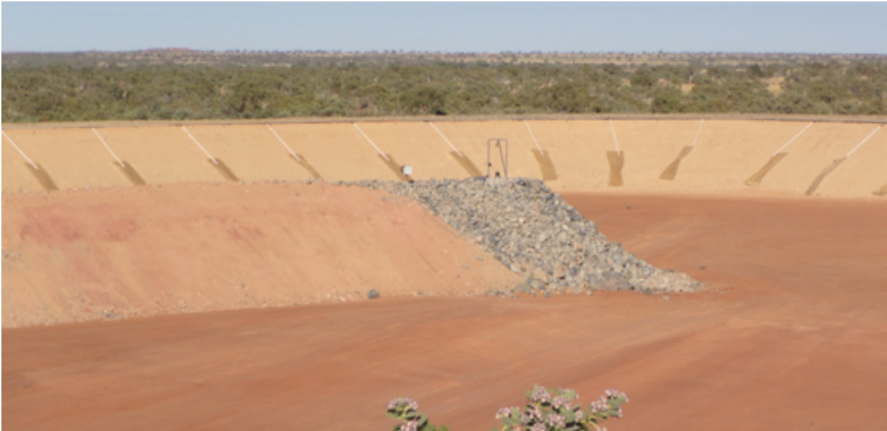
Completed Tailings Storage Facility
