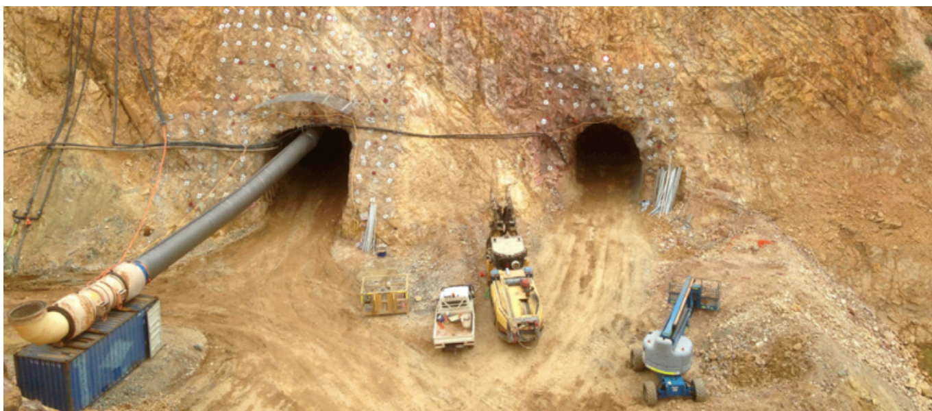
Underground development underway at Nicolson's
