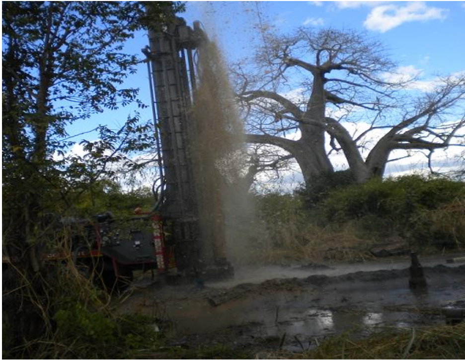
Figure 4 – Recently completed Water Bore Hole
