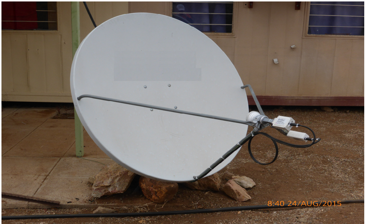
Ku Band satellite dish installed behind the main office at Lerala
