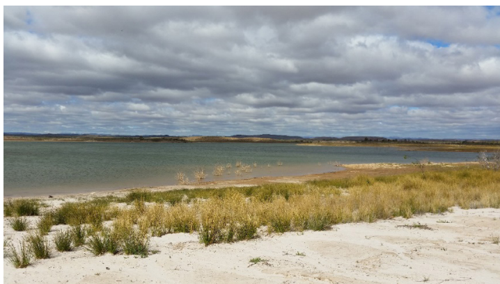
Figure 3: Retention Dam at Leigh Creek.
