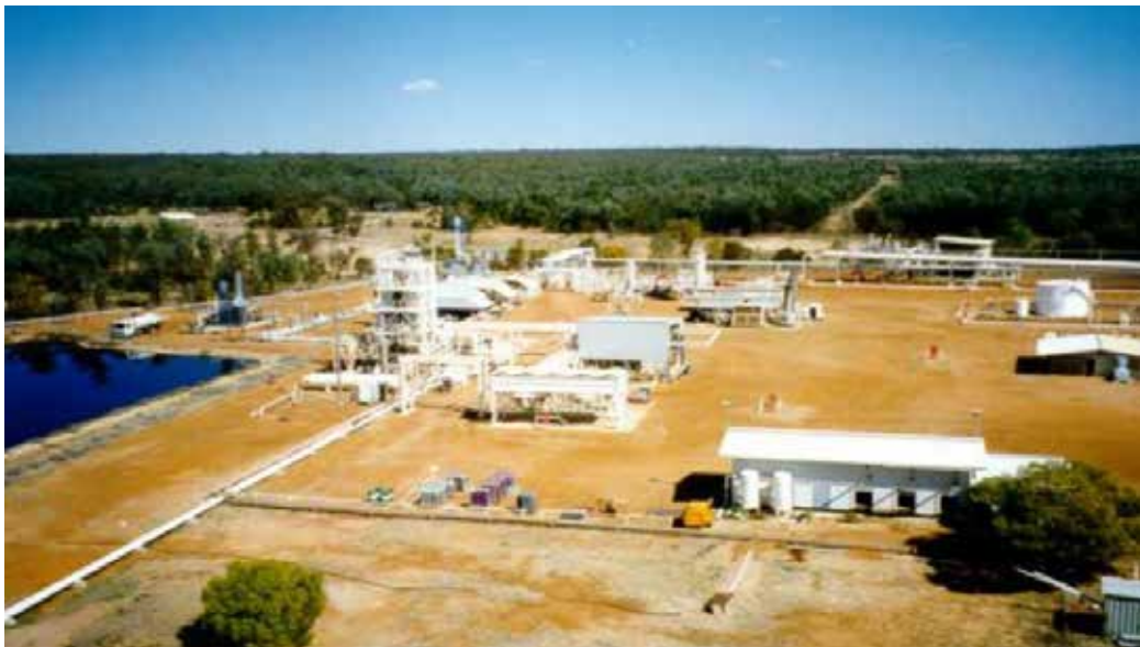
Figure 7-1 Kincora gas plant 1
