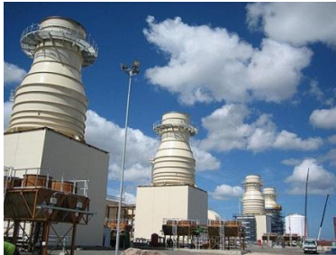
Open Cycle Gas Turbines
