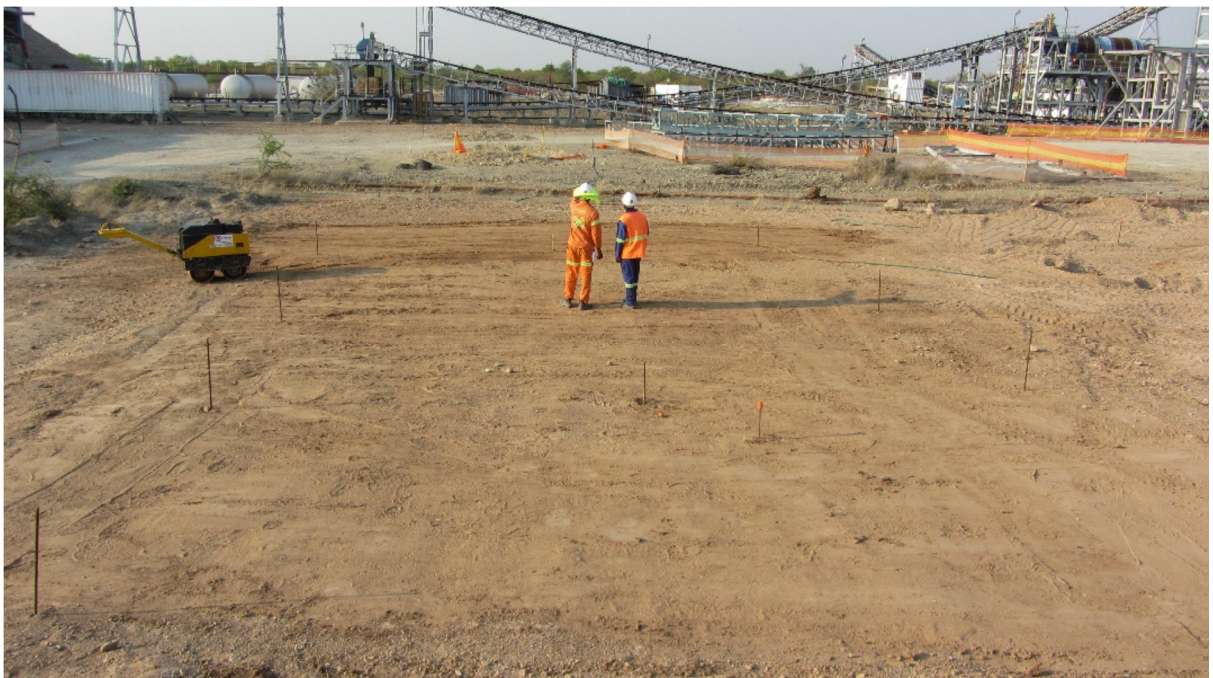
Secondary Surge Bin Module: Setting out and compaction of construction footprint
