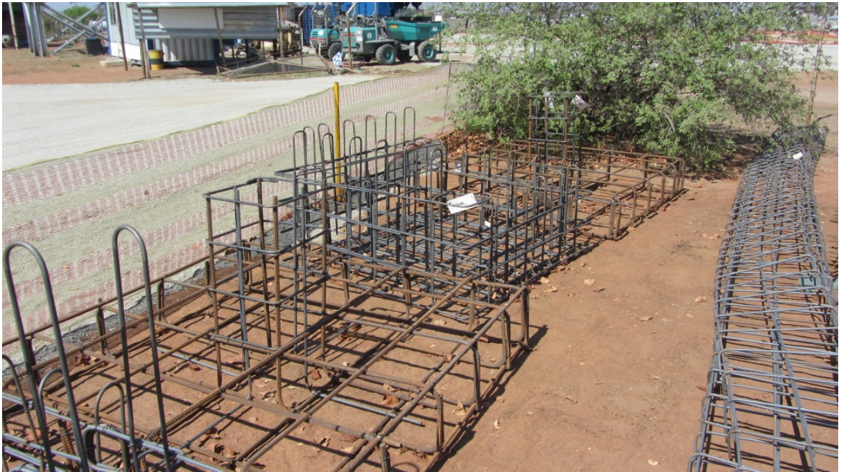
Rebar cages in preparation for concrete civil works
