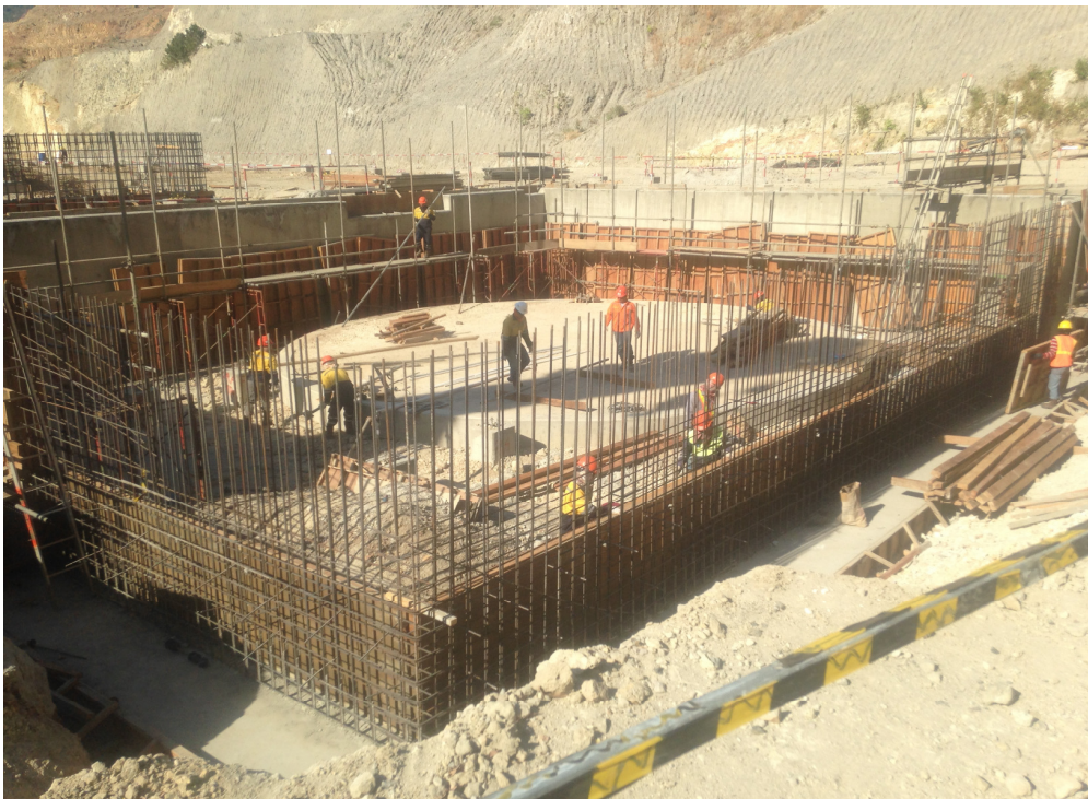
Image 4 – Foundations for the EW electrolyte circulation tank
