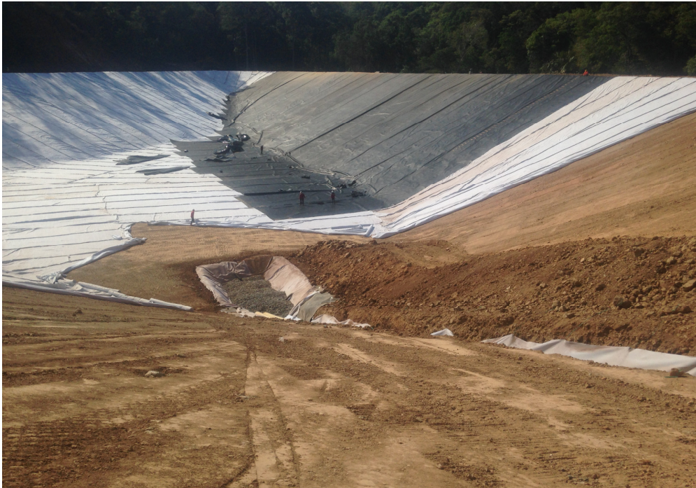
Image 3 – Lining of Stormwater Pond 2 commences
