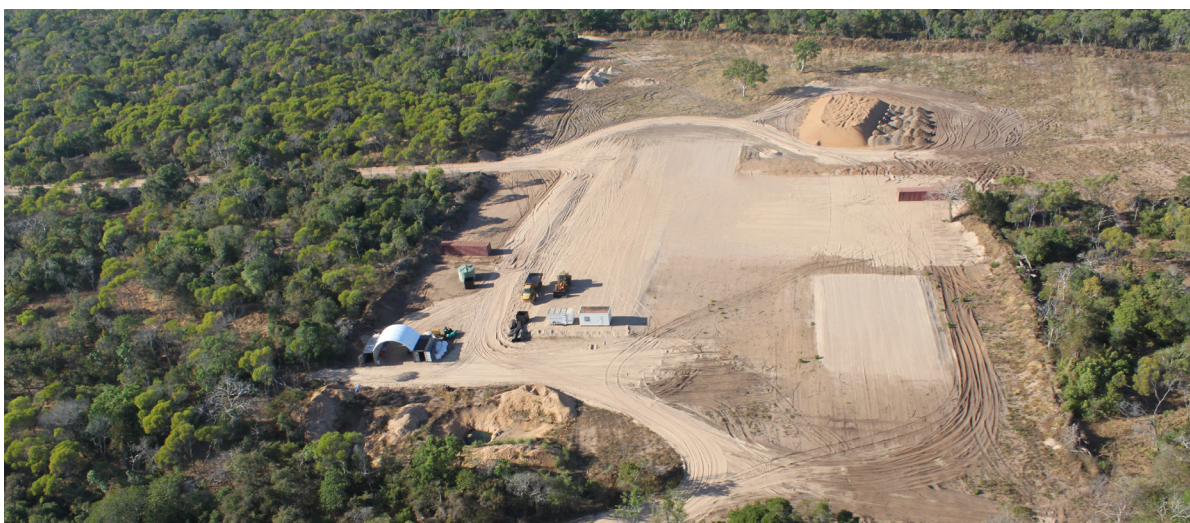
FIGURE 1: Civil works completed in preparation for the HMS processing plant with haul road from the initial mining area
