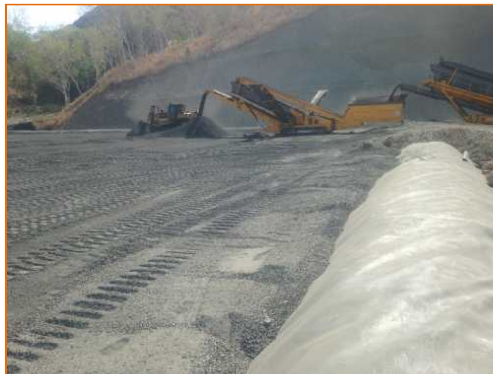
Crushing the bedding layer onto the KKV Heap Leach Pad
