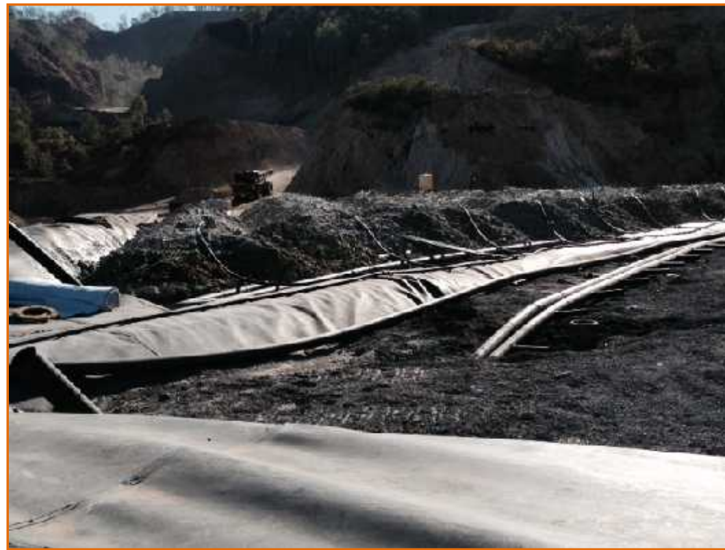
Raffinate Irrigation of Limestone
