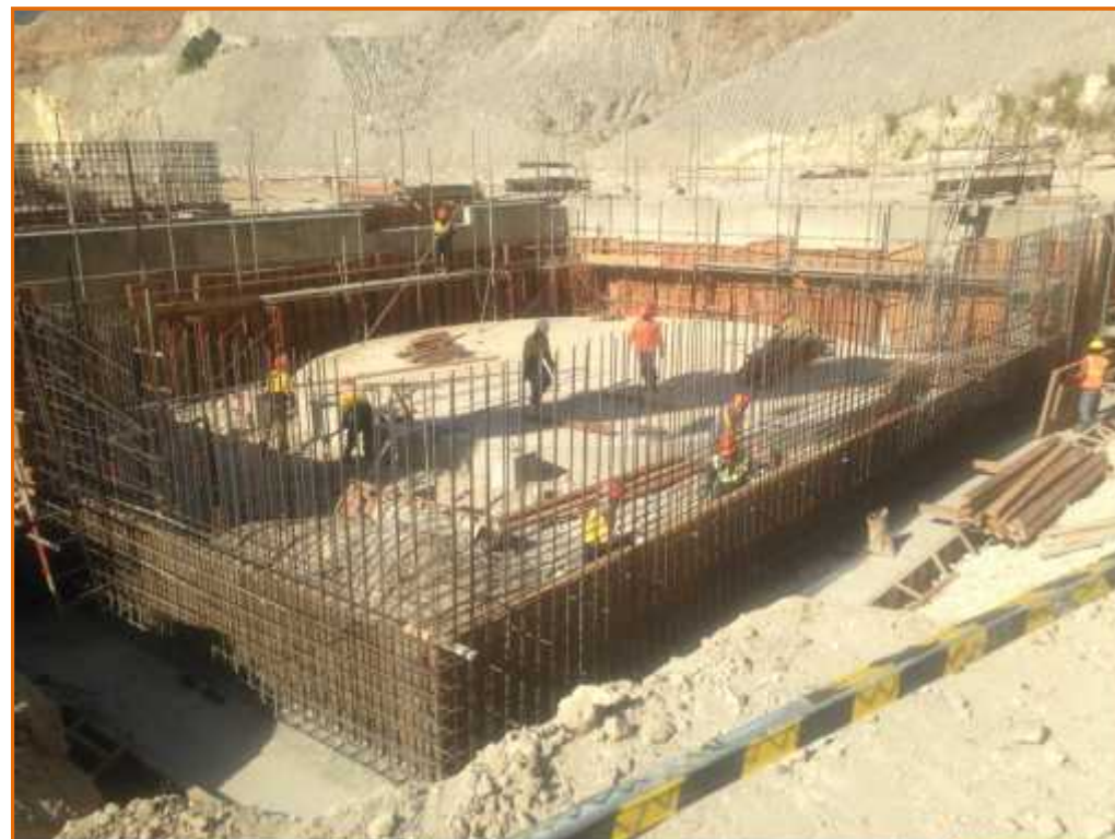
Concrete footings on SX-EW plant site
