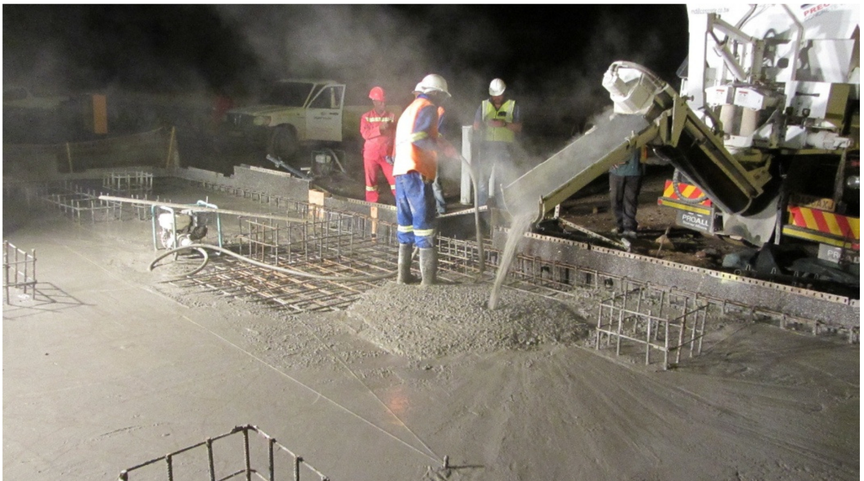
Area 102 (Primary Scrubber Module): Casting of floor slab
