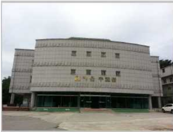
[the front view of South]
