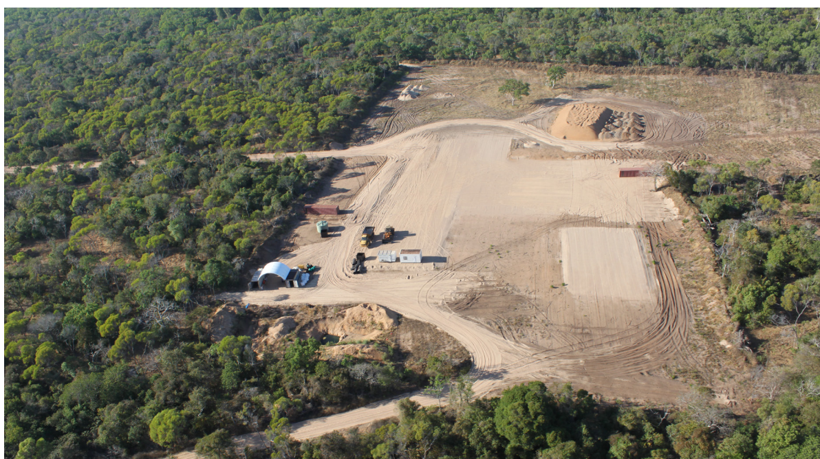
FIGURE 1: Civil works completed in preparation for the HMS processing plant with haul road from the initial mining area
