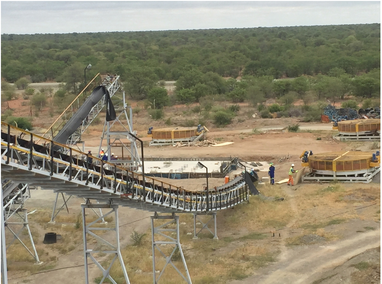
Figure 3: New concrete footings completed and ready for the erection of the new 400 tonne capacity DMS surge bin
