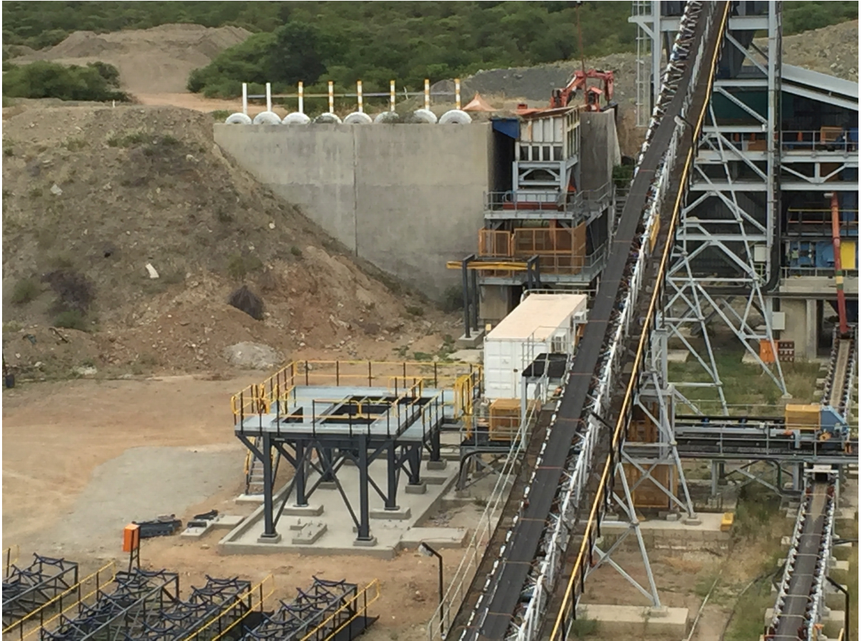
Figure 2: The new platform for the primary scrubber (left foreground) ready to accept the scrubber shell, the primary crusher (rear) and the refurbished conveyor (right foreground).
