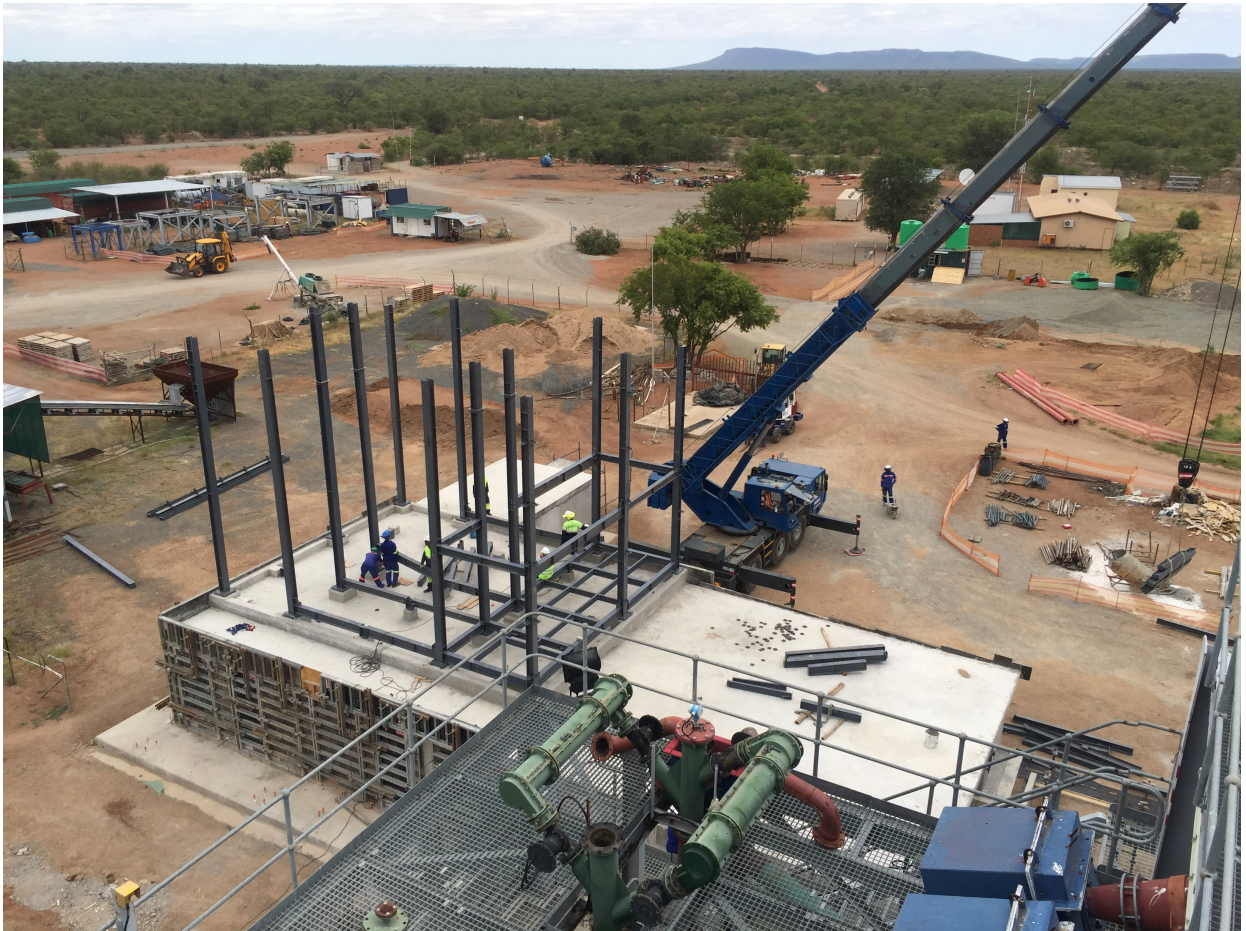
Figure 4: The newly-completed high-security concrete Recovery Module with erection of upper levels structural steelwork in progress.
