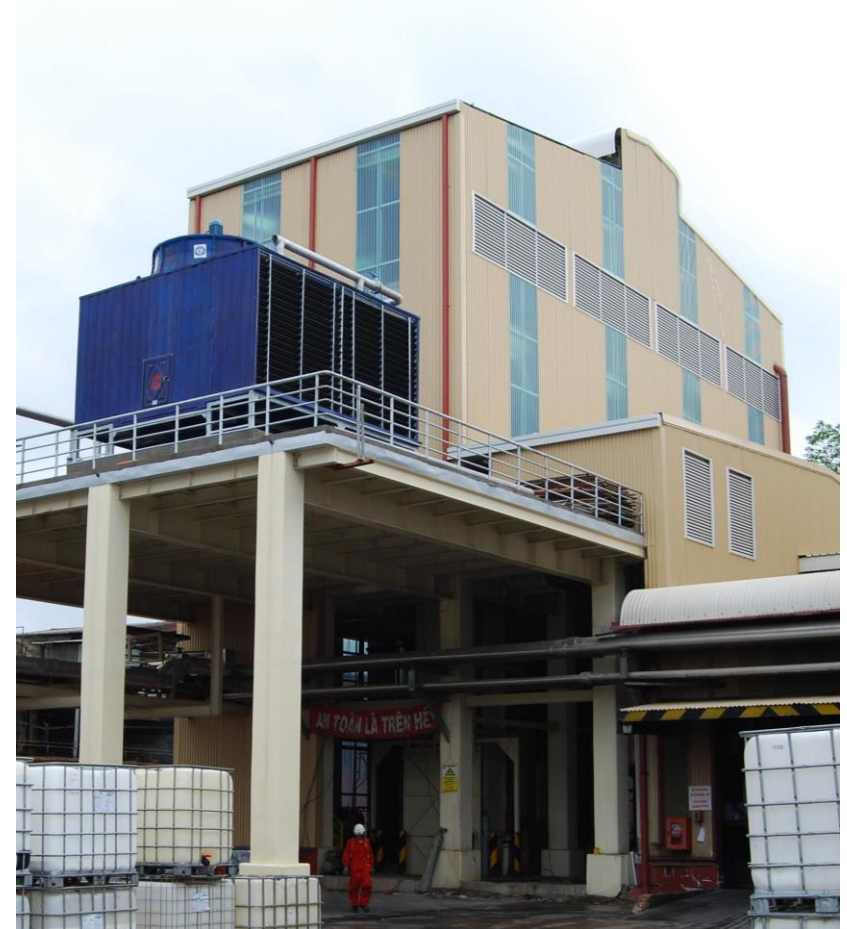
Nuplex Vietnam, Reactor building commissioned April 2013
