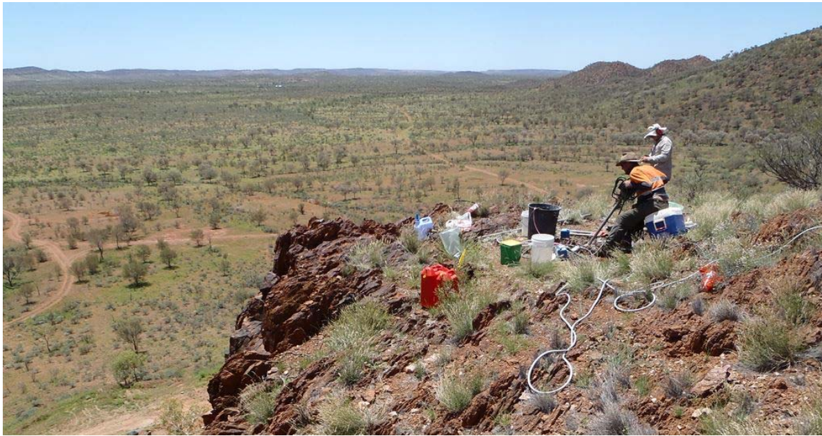
Figure 1 Hand held diamond drilling of the top part of the Rockface resource
