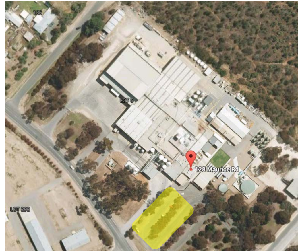
The proposed soft cheese plant (highlighted in yellow) will sit within the Murray Bridge site at 128 Maurice Road, Murray Bridge, South Australia.
