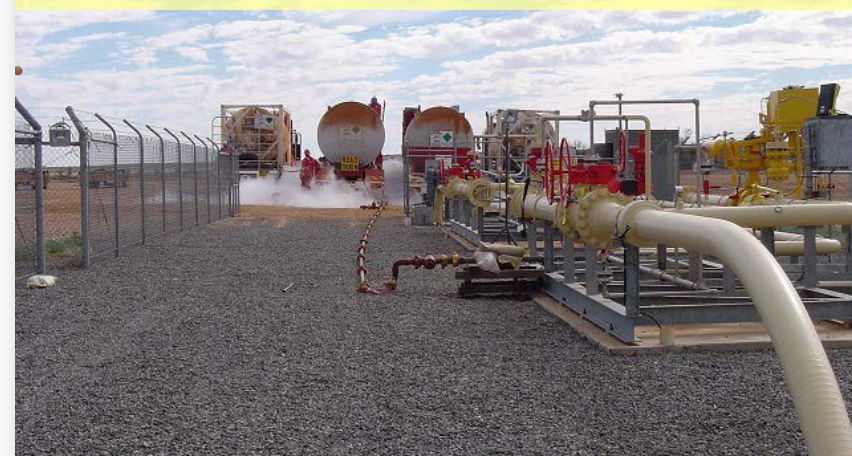
APA operates and maintains the Ethane Pipeline - Quarry View Scraper Station
