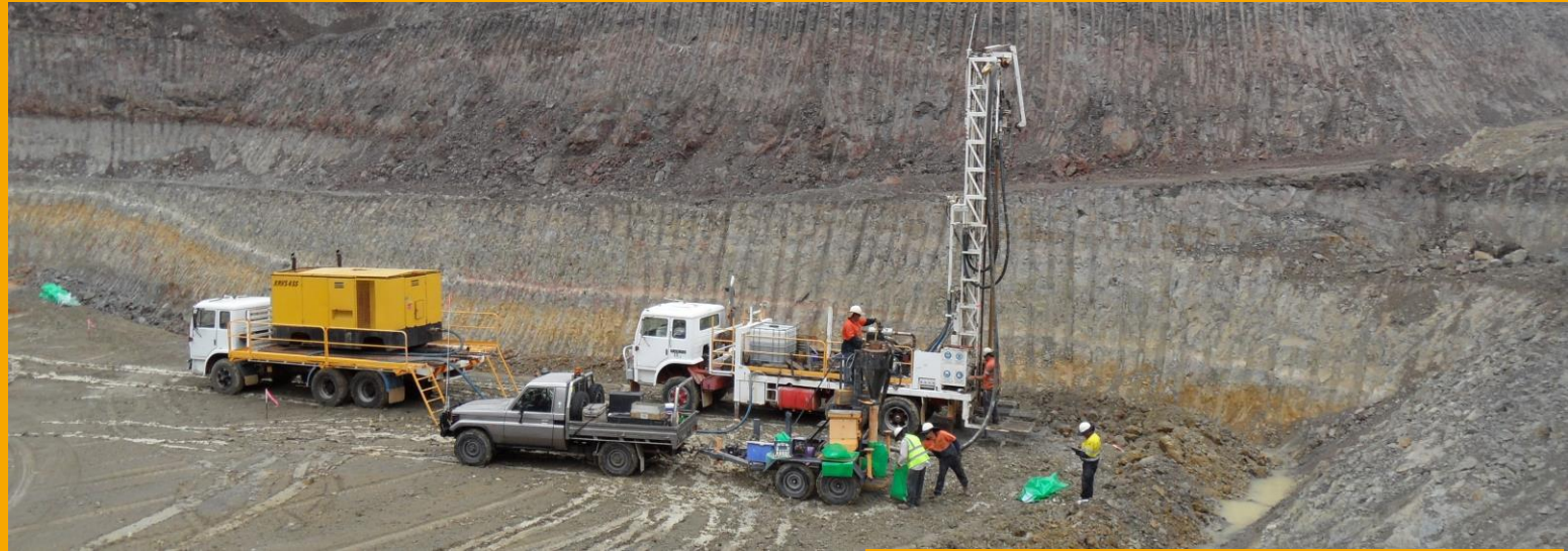
Geological drilling on the floor of the Portia open pit
