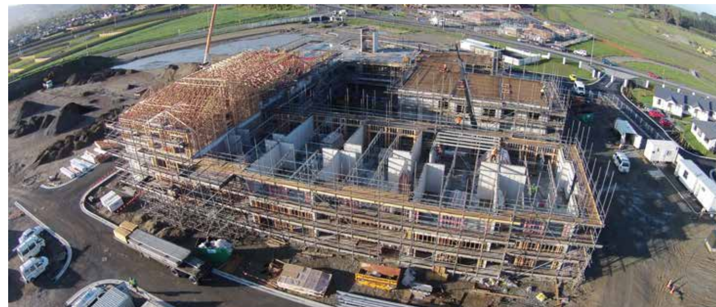
Summerset at Wigram under construction.
