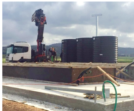
Modules installed onsite at Ha-Yogev municipal wastewater treatment plant
