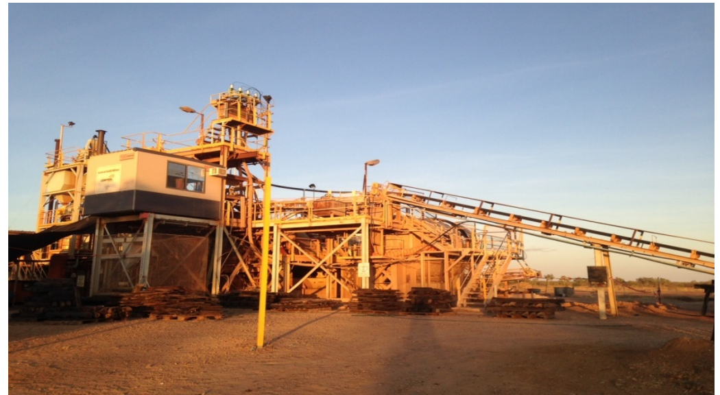
EOPL's Georgetown Gold Processing Plant
