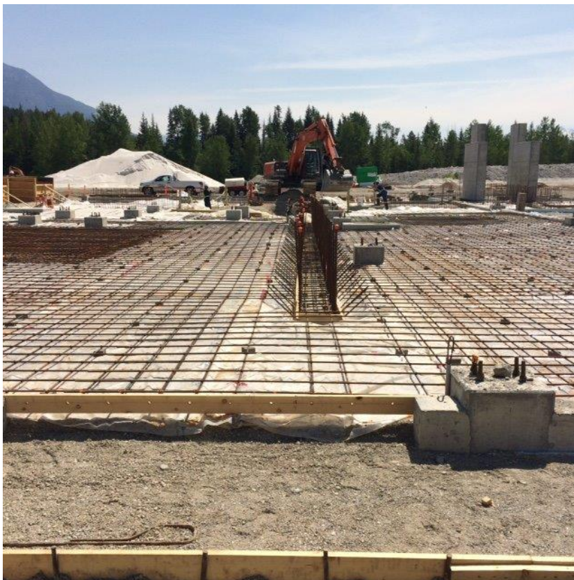
Process building floor slab preparation for concrete
