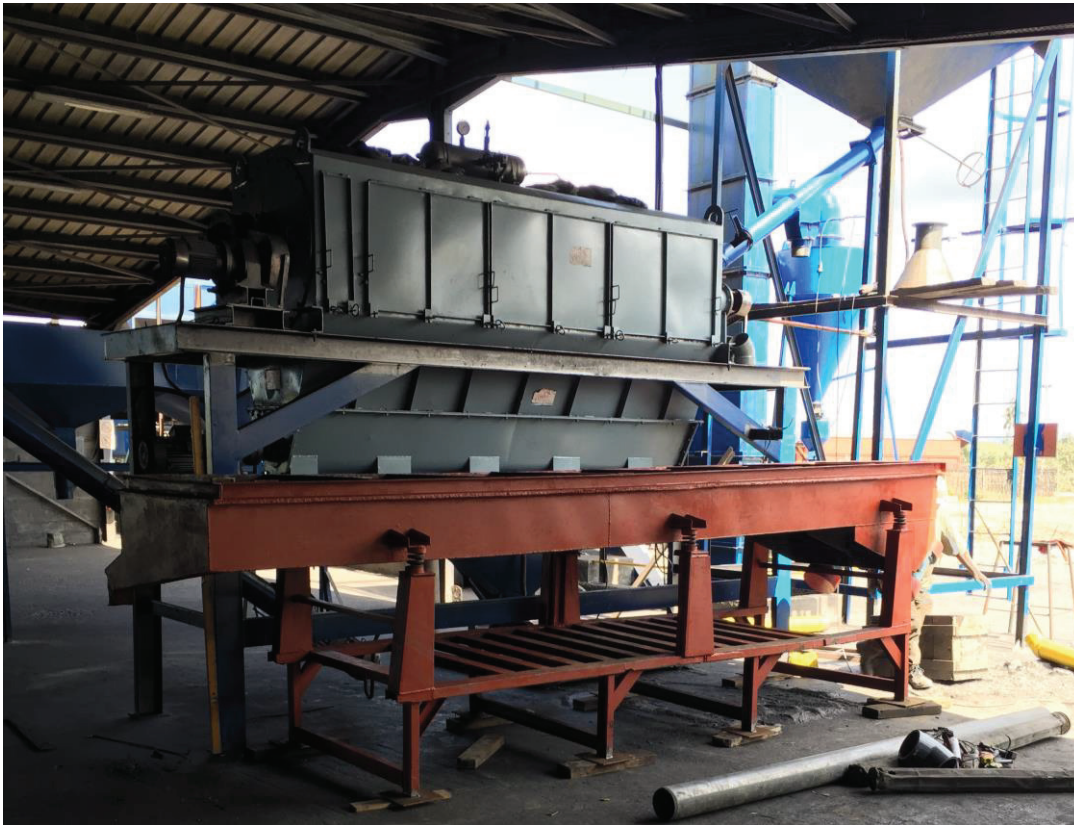
Vibrating magnetic separator being installed at Graphmada
