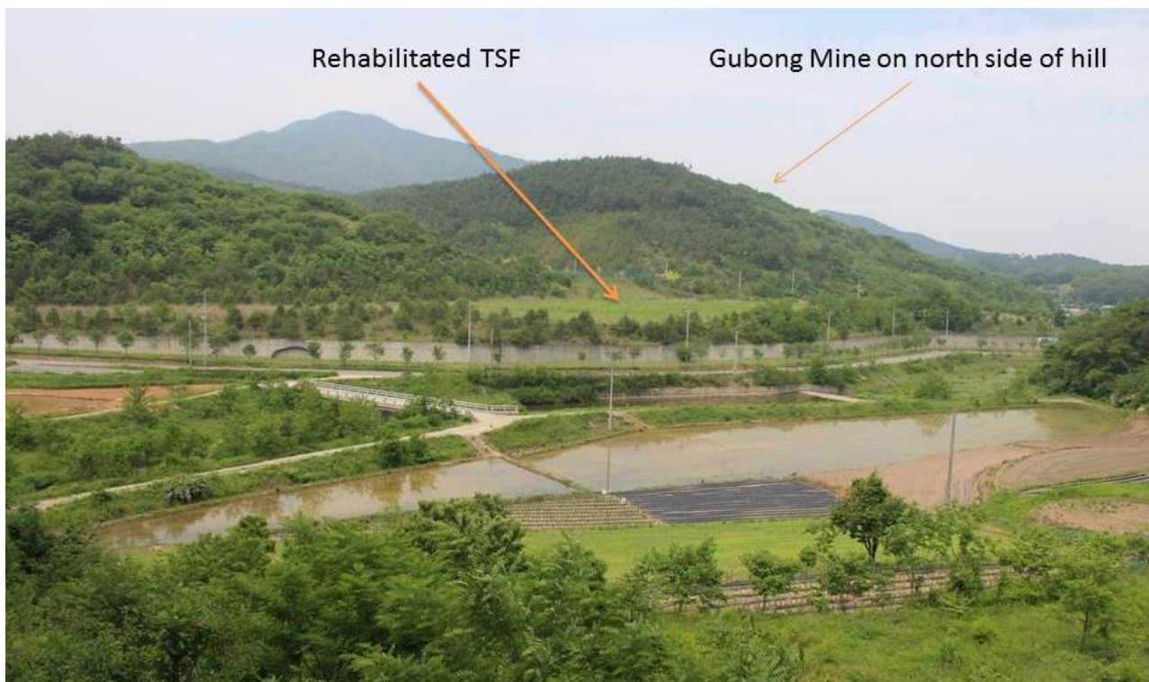
Photo 6: Rehabilitated TSF at Gubong
