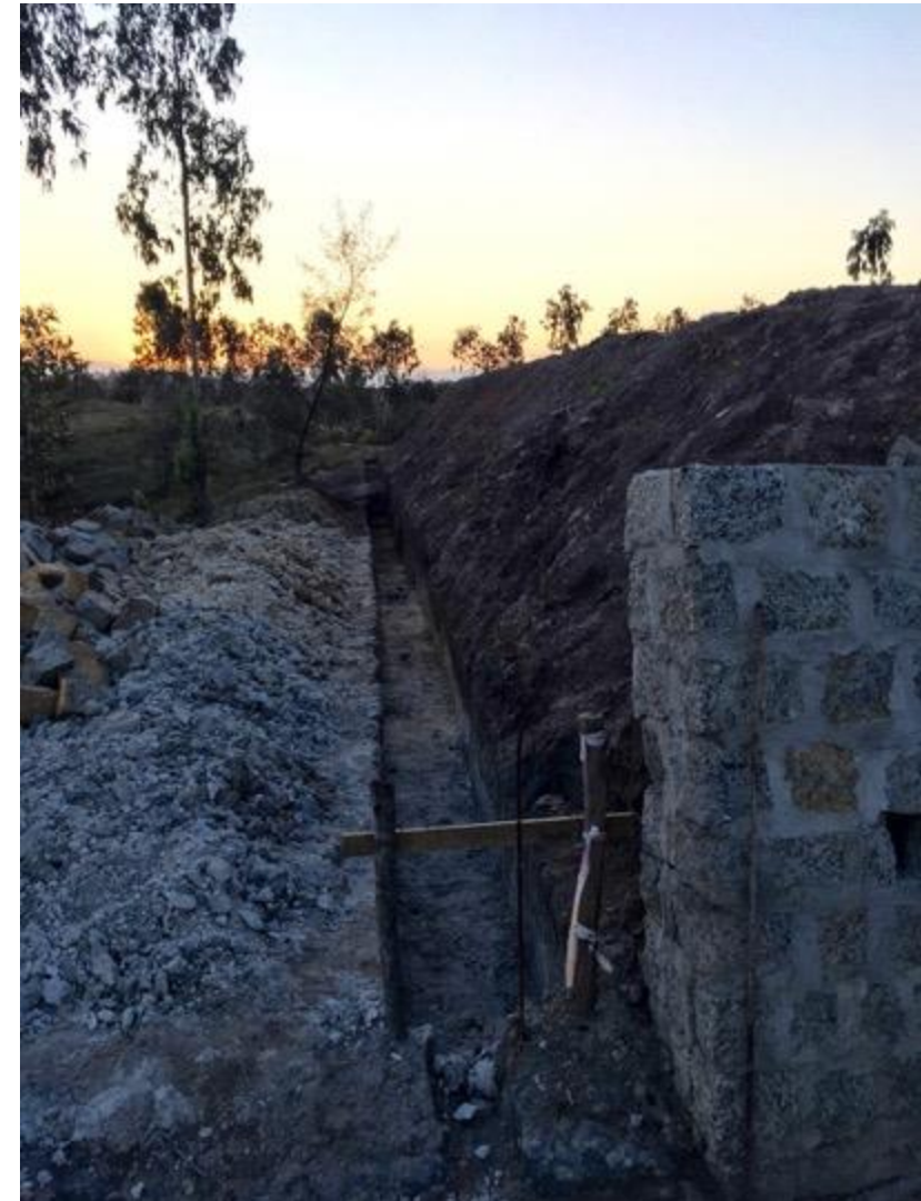
New Workshop & Stores retaining wall construction
