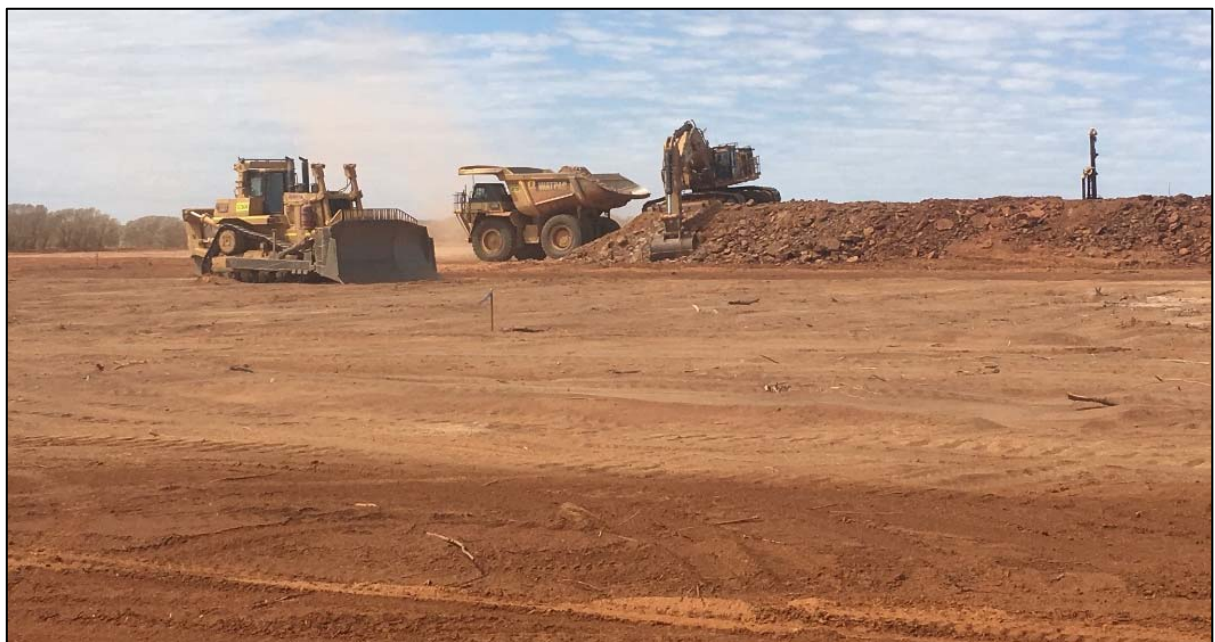
Figure 4: Blackmans open pit commencement
