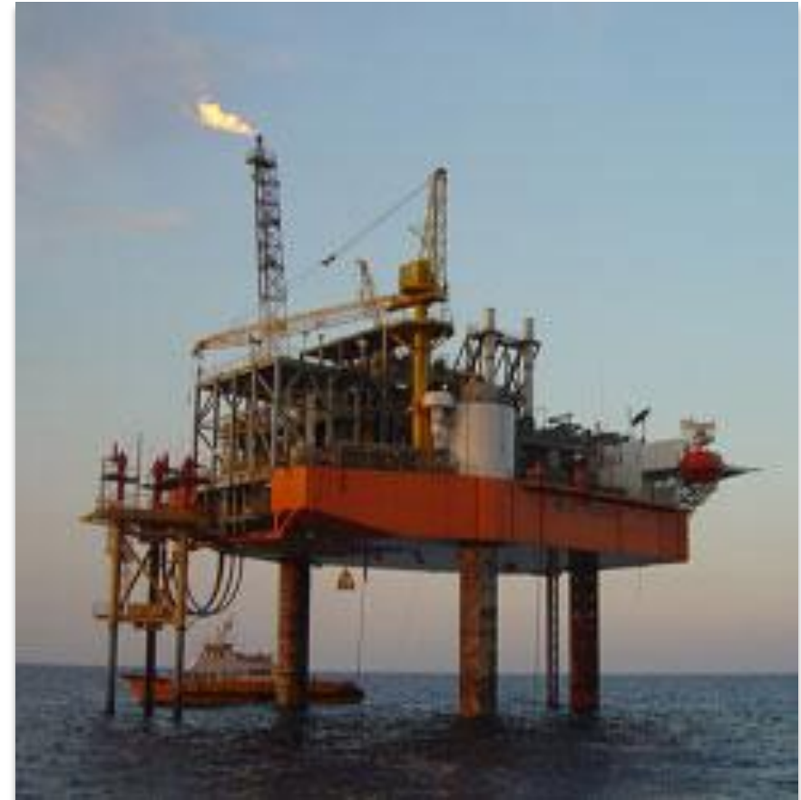
An example of a MOPU located next to a Well Head Platform illustrative of the CFS for the Loba Complex
