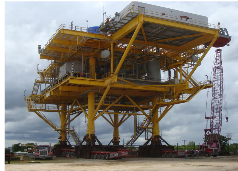
Example of processing facility for full field development of Lepidote Deep. This facility would sit on top of a jacket (not shown) next to a Well Head Platform
