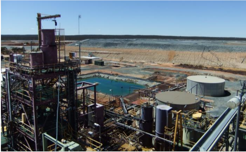
Mill with tailings dam in background
