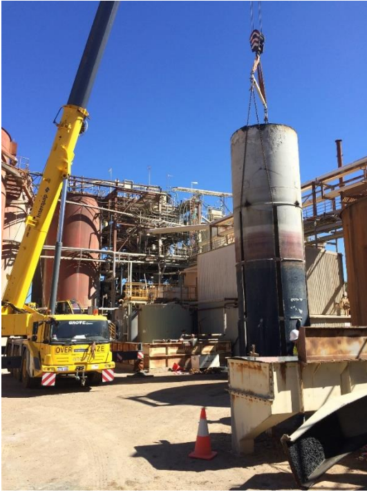
Photo 7: Final Leach Draught Tube Removed
