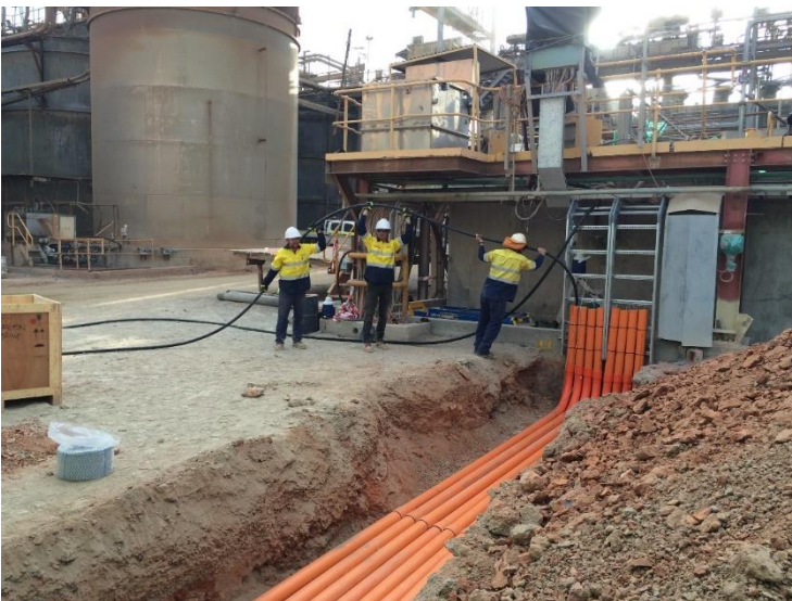
Photo 5: Running cable between Mill2 and MCC2
