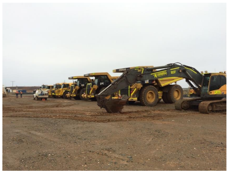
Photo 10: TSF Contractor's fleet mobilised
