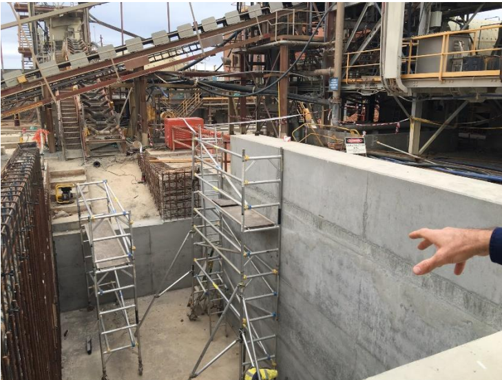
Photo 3: Mill 1 Feed Vault Repair
