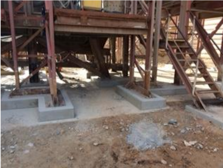
Photo 1: Repaired Crusher Area Footings
