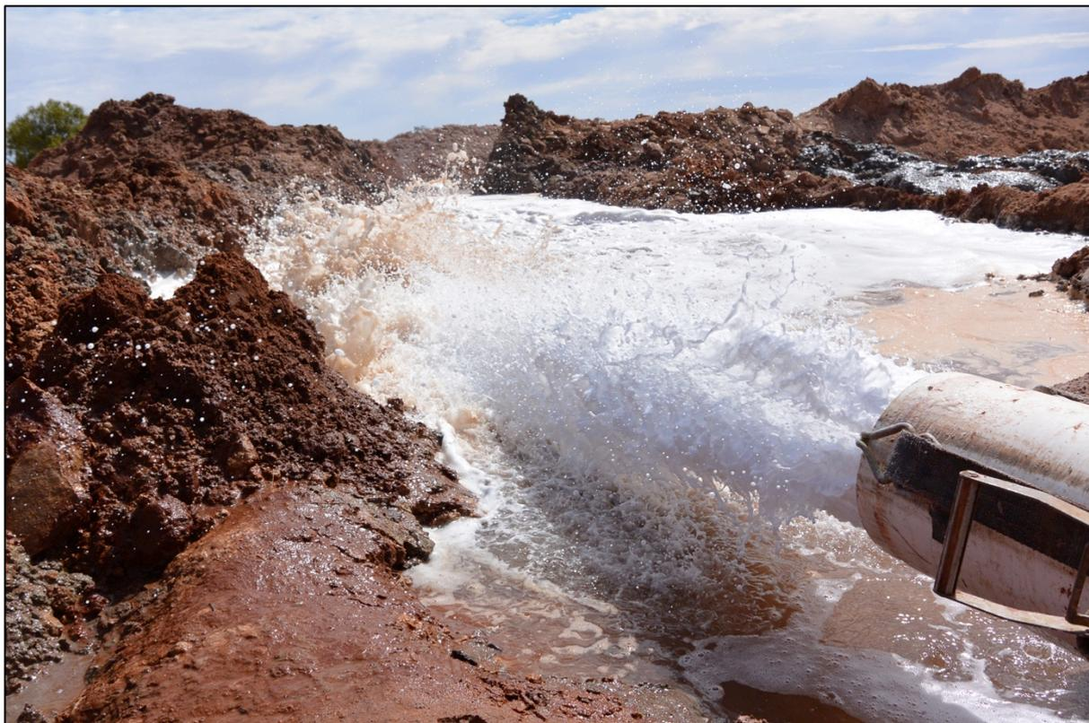
Figure 1: Airlift development has been completed on bores at Site A and Site B
