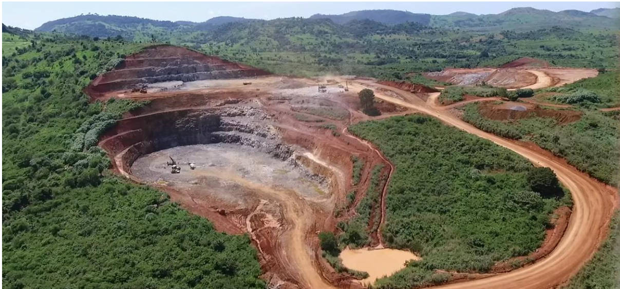
Antas Stage 1 open pit with Stage Two cutback and waste dump in background
