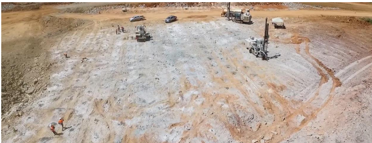
Antas Stage Two - drilling and explosive loading
