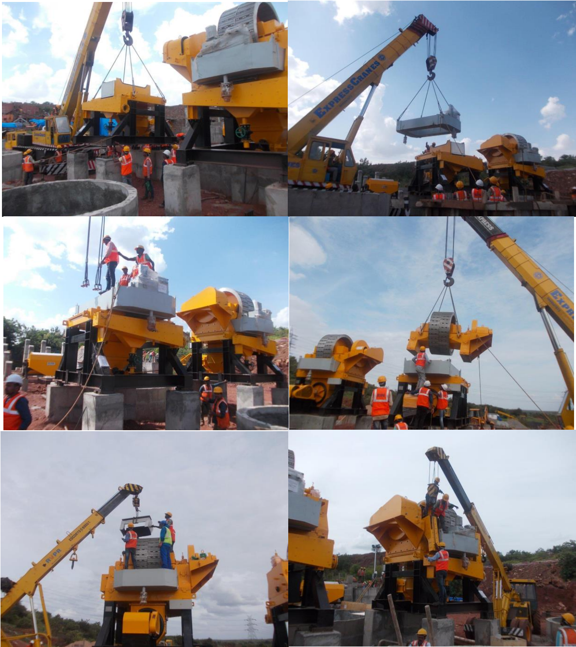
WHIMS Number Two Erection
