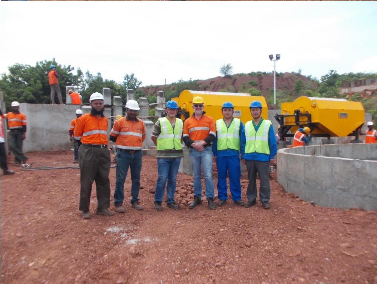
Completed LIMS Erection and the Team
