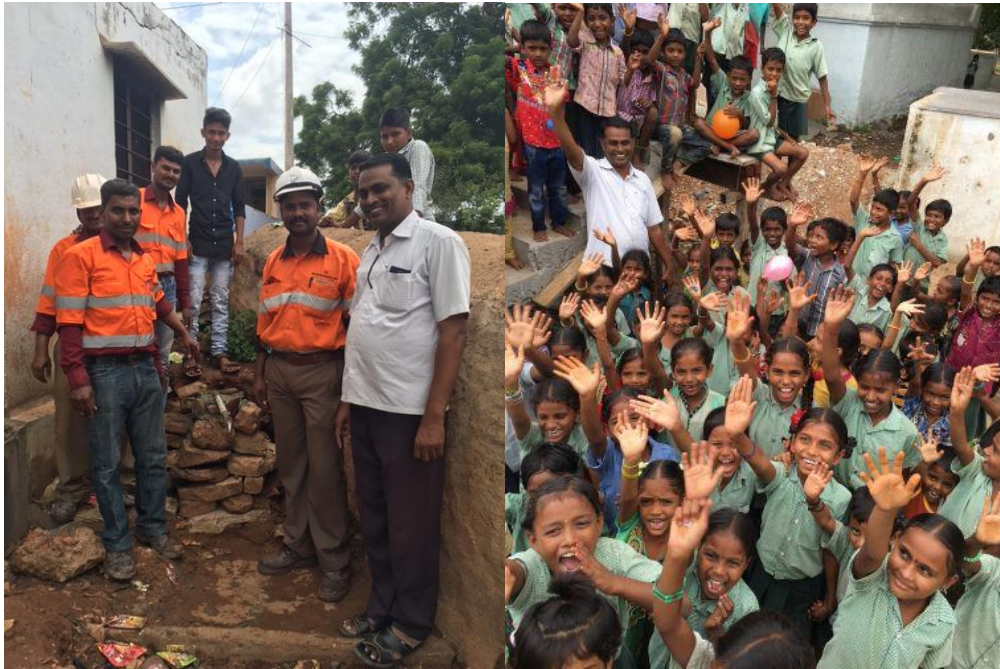
NSL Staff Repairing Water Pipes for Local School
