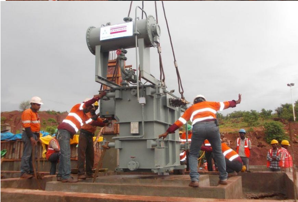
Transformer Erection
