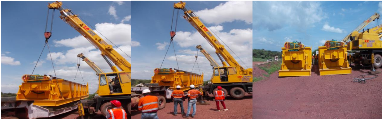
Equipment arriving on site
