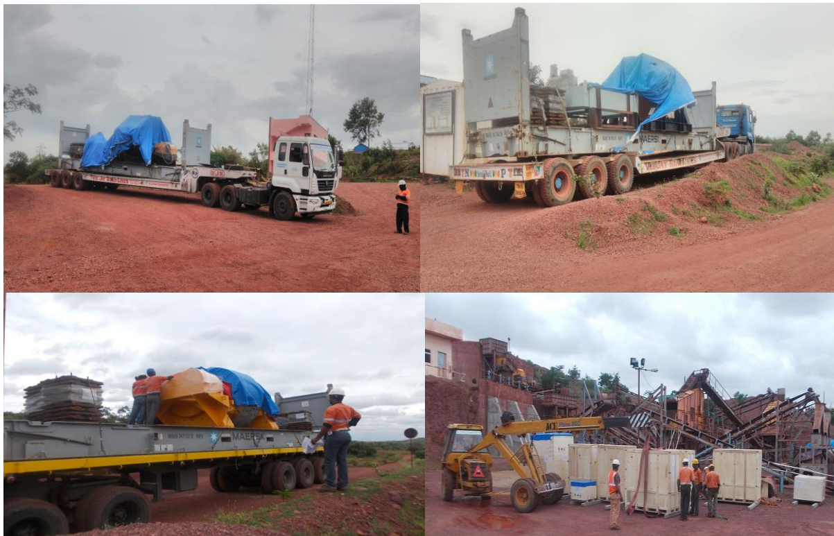
Equipment arriving on site
