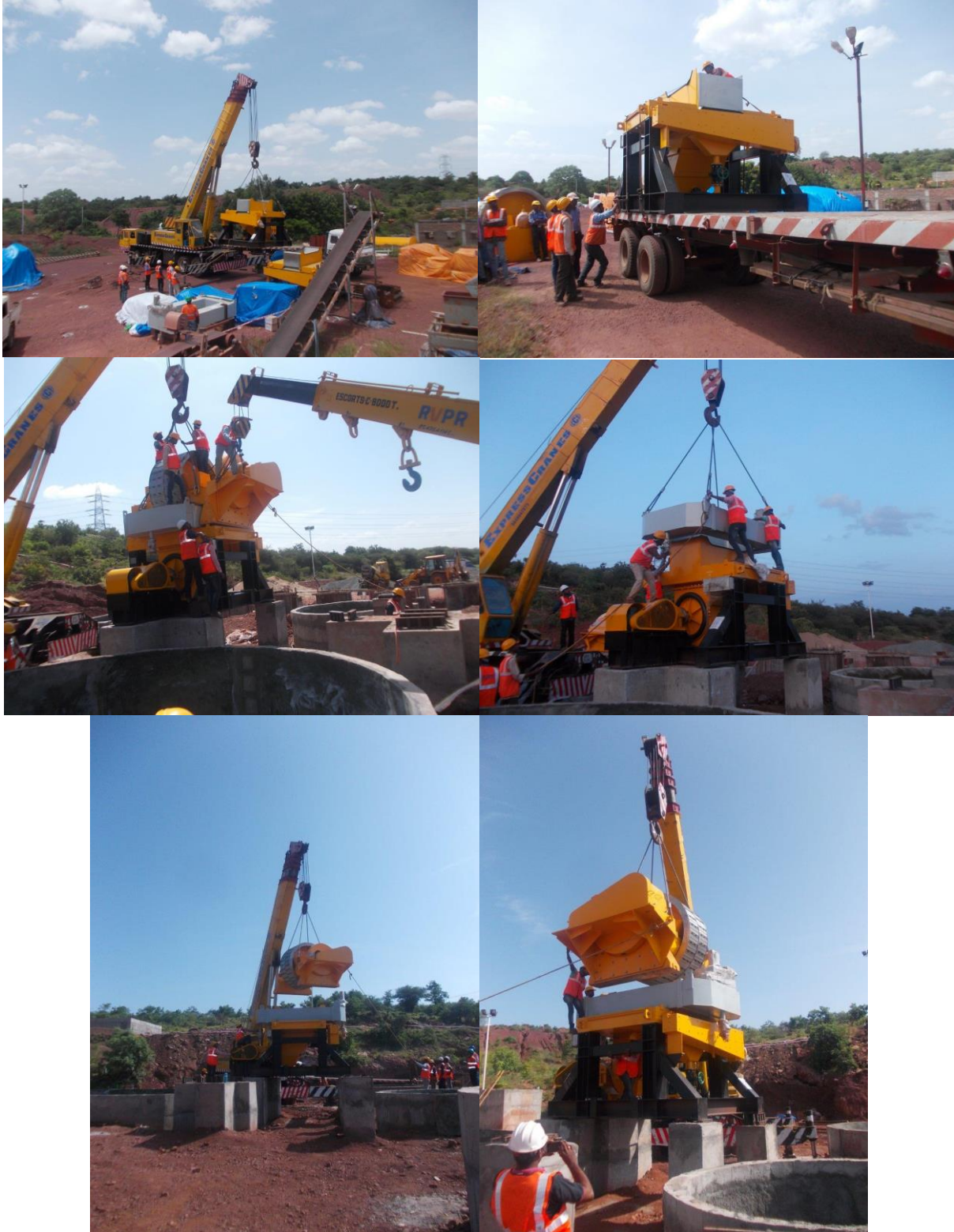
WHIMS Number One Erection
